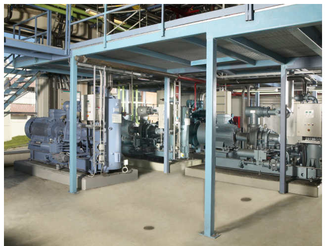
The picture shows a 2002 built -10°C machine room and four 1 MW Grasso screw compressors.
